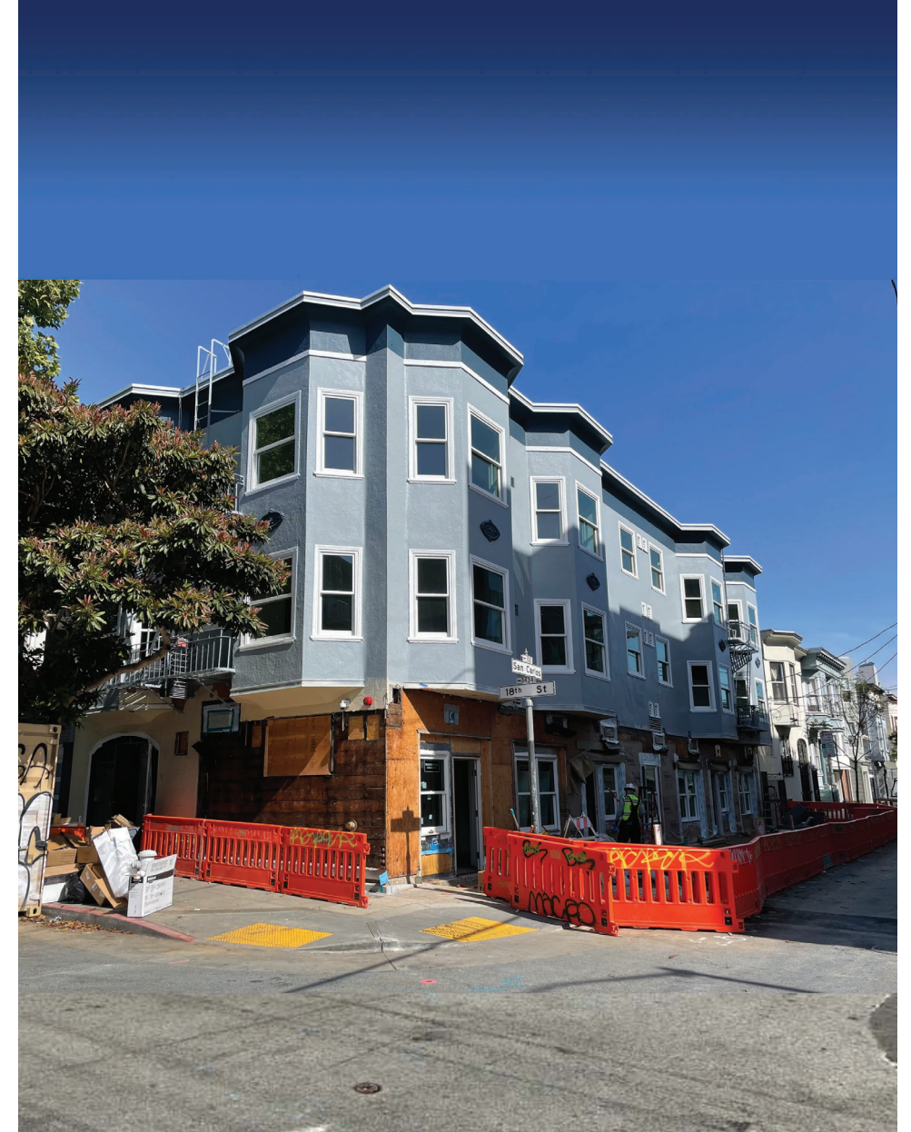
June.07.22 Construction Progress
